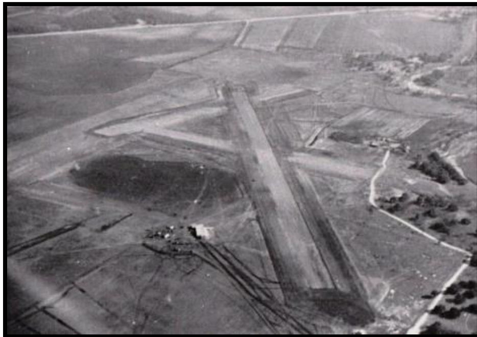
Photo: During Construction
