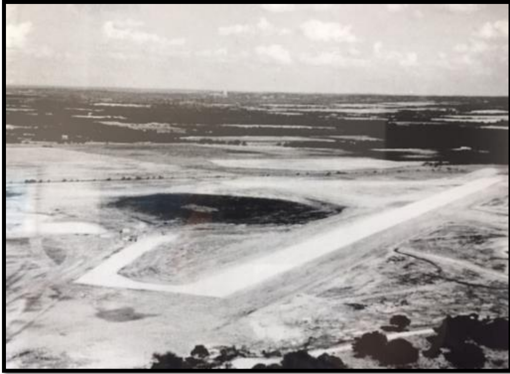
Photo: Construction Completed -1948
